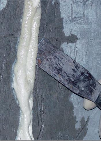
**For decades, chemical grouts have been the solution for sealing leaking cracks and fractures within sound substrates and the stabilization of unsound earthen materials.**
