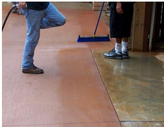
Efflorescence Removal Process with INCRETE JET PHOS
